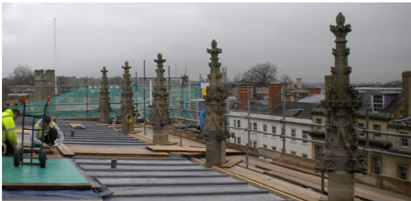
Roof works for St Mary the Virgin Church, High Street, Oxford
